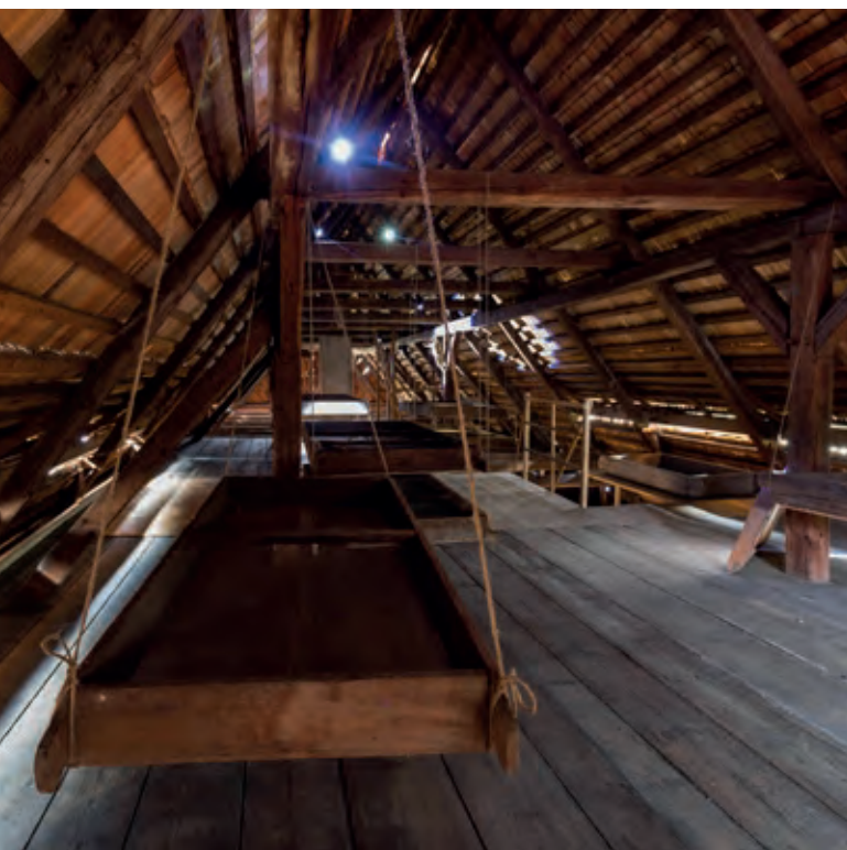
Tiers for drying hops in the loft of building of the exhibition Líska k sušení chmele na půdě expozice
